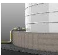
Insert a length of flexible pipe to absorb shocks & movements of pipe fittings from tank. Position the pipe directly on ground to avoid damage caused by standing over pipes.
