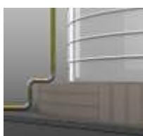
Tank overflow must be piped away from the tank to avoid undermining of tank base.
